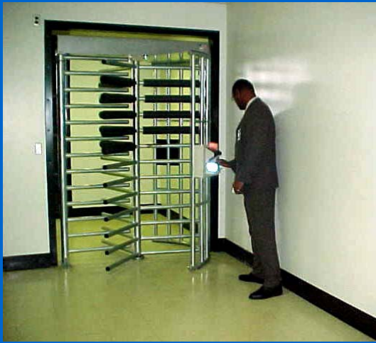
Turnstile Vestibule with Card/Hand Geometry Reader
